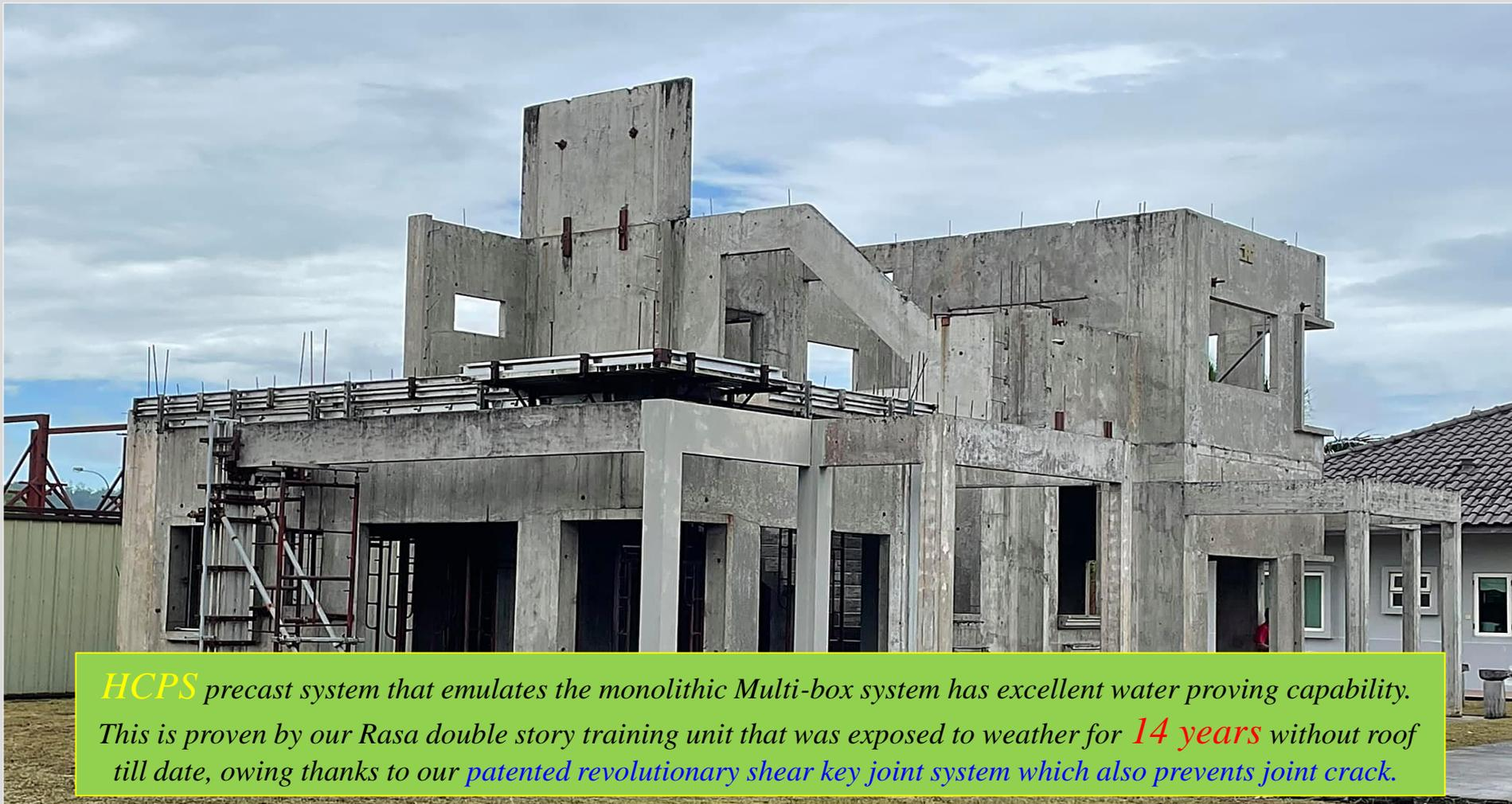
***HCPS*** precast system that emulates the monolithic Multi-box system has excellent water proving capability. This is proven by our Rasa double story training unit that was exposed to weather for **14 years** without roof till date, owing thanks to our **patented revolutionary shear key joint system** which also prevents joint crack.
